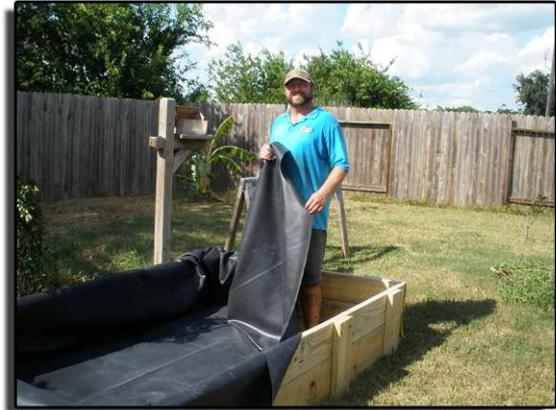
Now it's time to lay the liner into your frame. Make sure the liner fits all the way into the bottom edge of the framework, and leave a little extra slack in the bottom.
