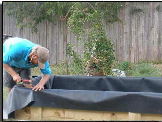
Staple the liner along the top edge of the framework to secure it while you finish it off.
