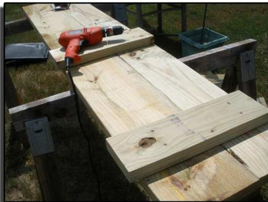
Secure treated 2"x12" to either another 2"x12" or a 2"x6" using sections of 2"x6" braces spaced 2'-3' on center. Fasten with wood screws.
