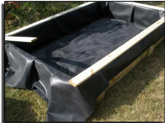
Now you can screw treated 1" x 4" boards on the top of the liner and framework. This will give you a finished look.
