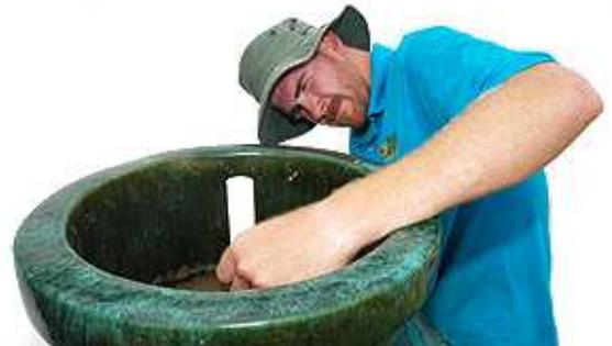
12. Thread the tubing through the cracks of the grating and slowly lower the piece into place. Once in place, level the pot using shims. Shims should only be placed directly over the thick supports in the grating to avoid sagging and shifting.
