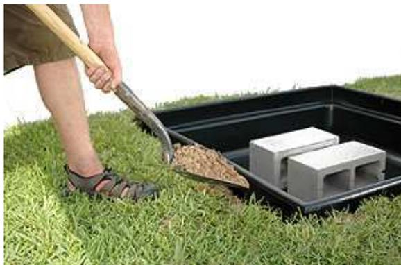
5. Place 2-3 cinder blocks (depending on the piece) in the middle. For light pieces place the grating on top of the cinder blocks. Heavy pieces require several cinder blocks and must sit directly on the blocks with the grate cut away to go around the piece.
