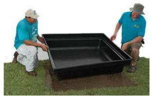
3. Backfill soil around the box packing in firmly.
